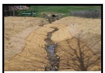
Matting 4) Once all the matting is laid out and secured with stakes, cover trenches with a few inches of soil, tamp it down and lightly cover top edge with straw to undisturbed landscape.
