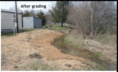
Option 3: A stream site in Newland, NC. The landowner's home is less than 20' from the water with 2'-3' vertical banks (above left photo). Above right photo shows newly graded, stabilized and planted bank.
