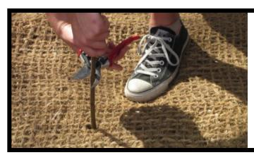
Step 2: Orient livestake with leaf buds facing upward (pointed end goes into the ground). Hand push or gently hammer livestake ¾ of the length into the bank. Make sure to leave 3"-4" sticking out of ground above soil line. If the top of the stake is smashed, make a clean cut for faster and healthier healing of the livestake.
