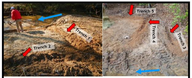
Blue arrow depicts water flow direction. Above left photo shows a site with Trench 1 perpendicular to the stream at the beginning of mat roll. Trench 2 is to secure top of mat. Above right photo depicts a site where another matting layer is needed due to typical high flows. Trench 3 and Trench 4 are dug perpendicular to the stream for start of rolled matting. Trench 5 is parallel to the stream at the top of the bank.
