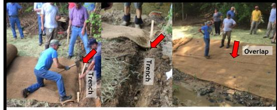
Matting 1) Lay start of matting in trench and tamp in 2' oak stakes with nail on end. Add every 1.5' to top of trench. Overlap extra matting rolls by 1'.
