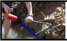
Step 1: Within the first 12" above the current water level, angle the metal rod perpendicular to the bank. Hammer a pilot hole and pull metal rod back out after starter hole is made. Livestake will go in starter hole; perpendicular to the bank.
