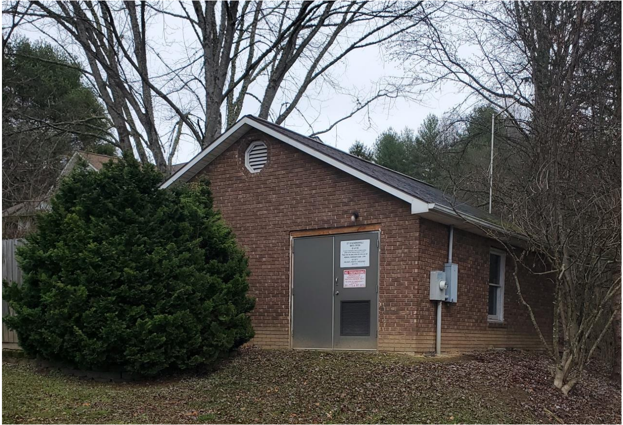
Site 119: Mountain Valley Hydro 15 Pumphouse Rd Approx. 8 Squares
