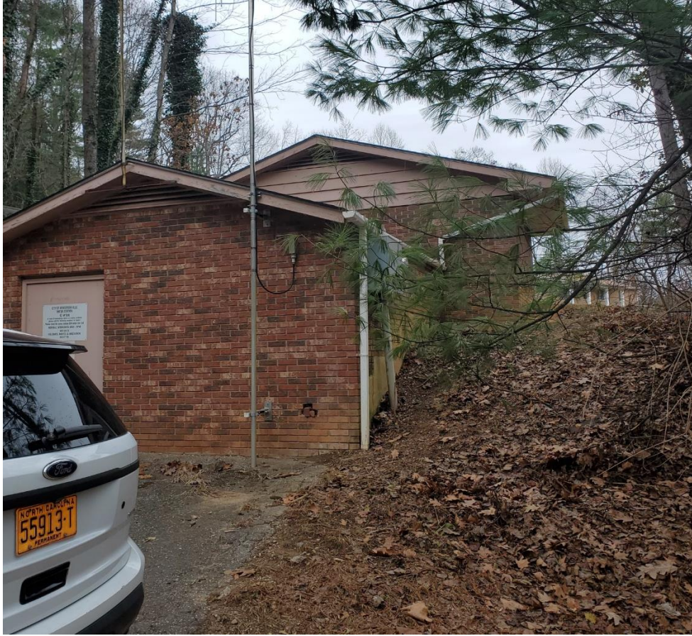
Site 106: Dellwood Hydro 907 Greenwood Dr Approx. 8 squares
