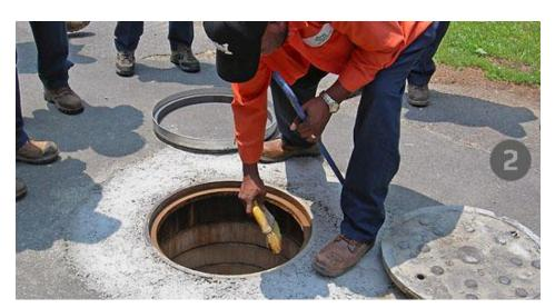
2. Remove all buildup on surfaces the Manhole Riser touches.
