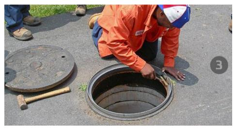
3. Expand linkage until the Manhole Riser is tight. That's it.
