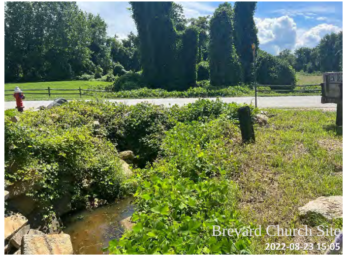
Photo 8 – Looking upstream at UT3 restoration reach (across road)
