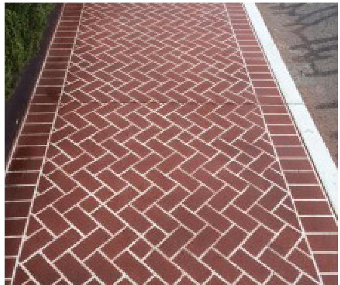
Brick Patterned Sidewalk | Wespray On Paving
