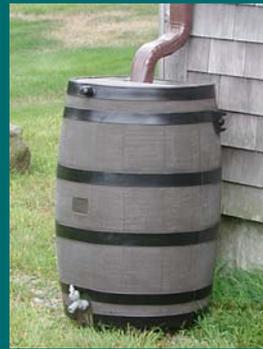
Rain barrel – an example of a technique for capturing rainwater
