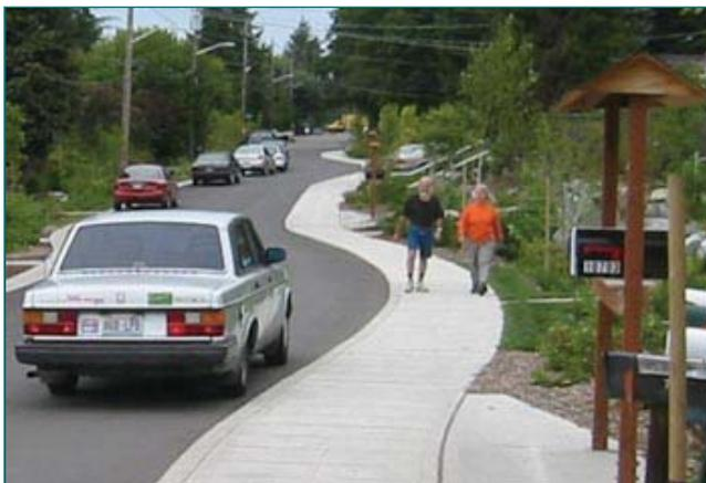
“Park Street” example: This Seattle street has been transformed by narrowing the pavement and replacing portions of the former roadbed with rain gardens
