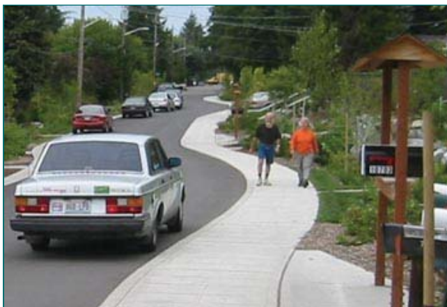
“Park Street” example: This Seattle street has been transformed by narrowing the pavement and replacing portions of the former roadbed with rain gardens Source: City of Seattle Public Works
