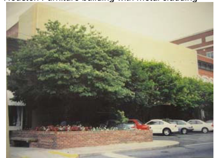
Houston Furniture building with metal cladding
