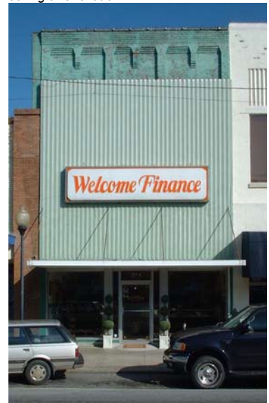
The brick corbelling of the historic façade is still visible above the metal skin applied during a renovation.
