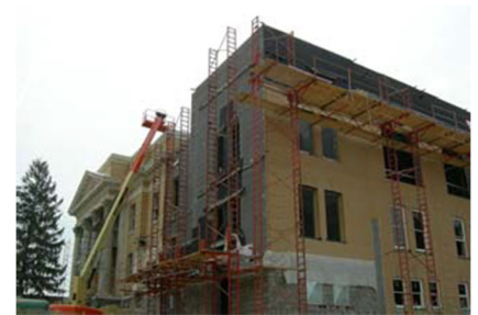
Exterior materials and design for the Historic Courthouse addition are compatible with original design.
