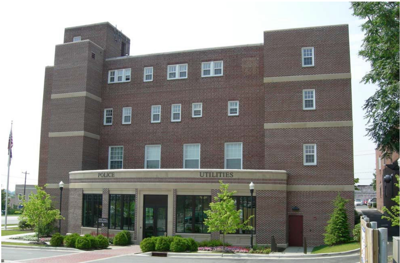
A recent City Hall rehabilitation project, which was completed in 2005, included a major addition to the rear of the building along Sixth Avenue East.
