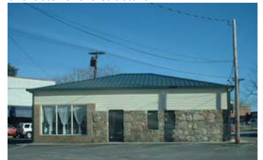
Over the course of several renovations, different exterior materials were used without consideration of the original character of the structure.
