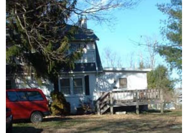
This deck is easily seen from the street and lacks a level of detail consistent with the structure.
