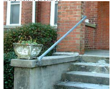
Metal pipes and fittings were often used in retrofit situations for railings but are not historically accurate and detract from the otherwise fine craftsmanship on many historic structures.
