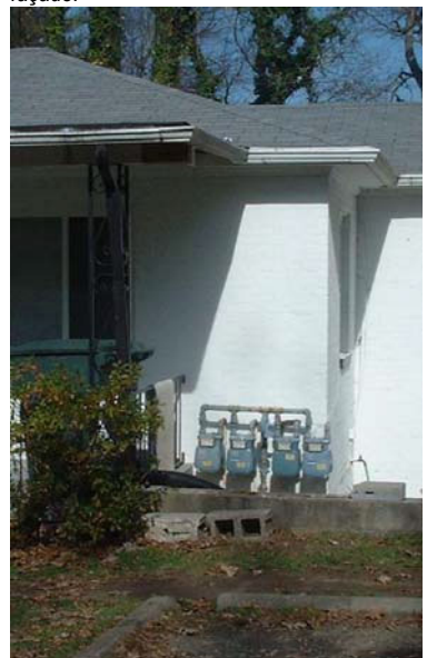
The utility meters should have been located on the side wall rather than the street façade.
