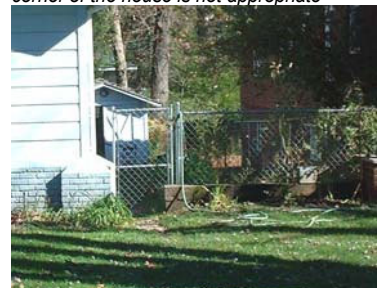
The use of chain link fencing at the front corner of the house is not appropriate
