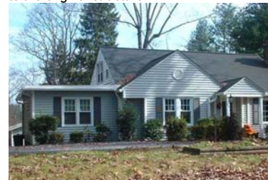
The addition on this home would have been more successful with a roofline that related to the original structure.
