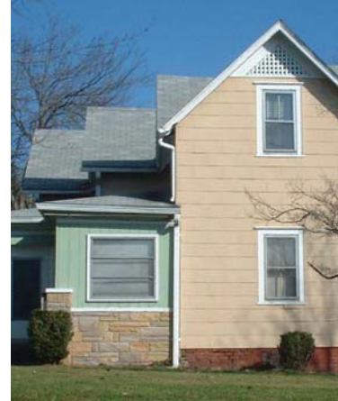
The siding material and windows on this addition are not appropriate for this building.
