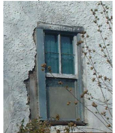
The stucco on this small cottage has been neglected and now the wood structure is exposed to the elements.
