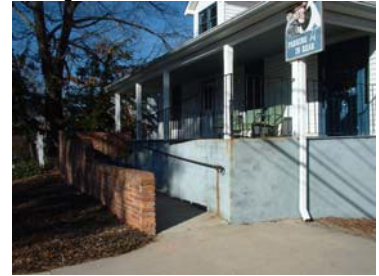
This ramp dominates the front façade and uses materials that are not in keeping with the original structure.
