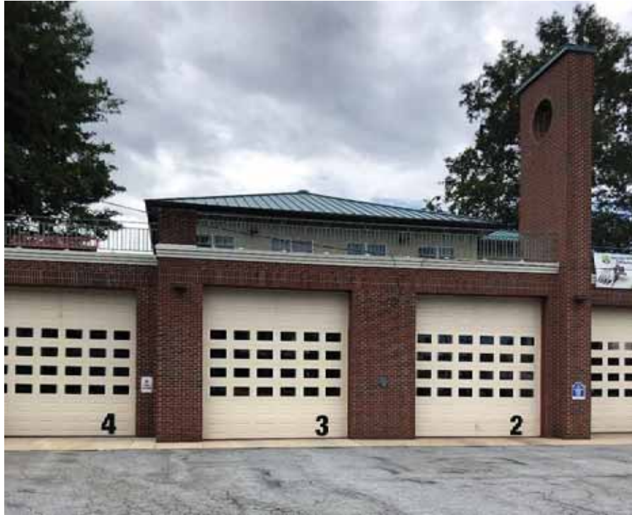
Photo 1 – Rear of Fire Station
