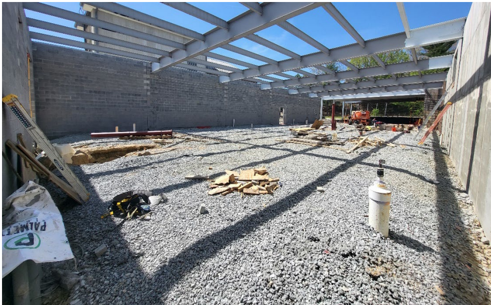
Biosolids Thermal Dryer Facility Construction. April 2026.
